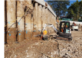
Ground water drainage being installed between piles.
