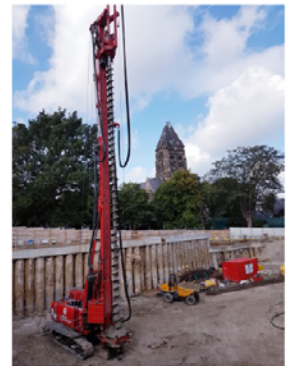
Bearing piles in progress.
