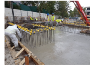
Construction of external retaining walls in progress.
